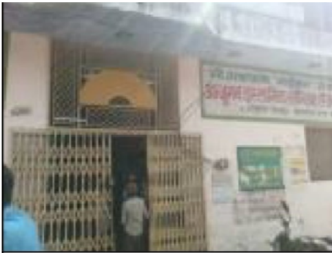
Building Front View
