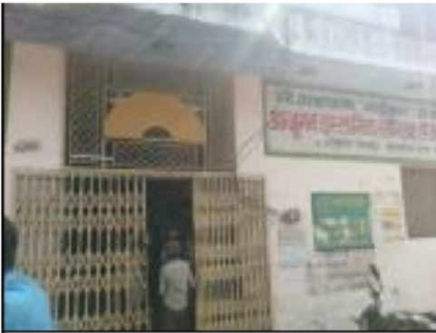
Building Front View
