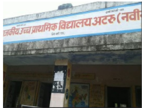
Building Front View
