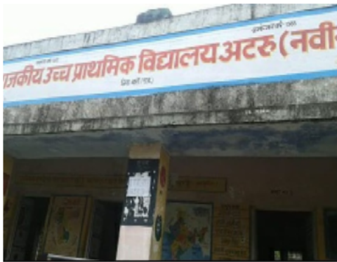
Building Front View
