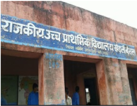
Building Front View
