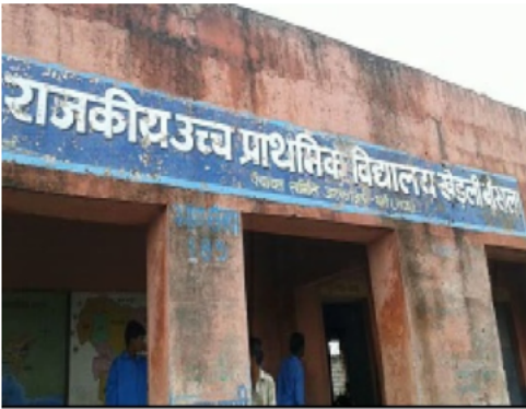
Building Front View
