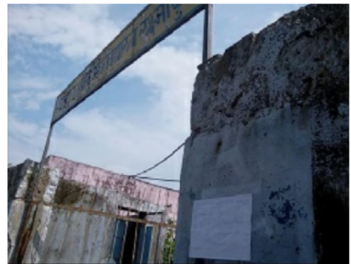
Building Front View
