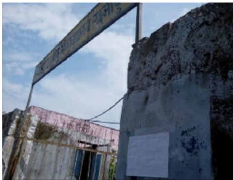
Building Front View
