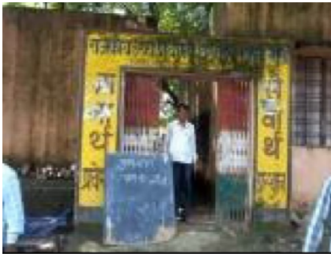
Building Front View
