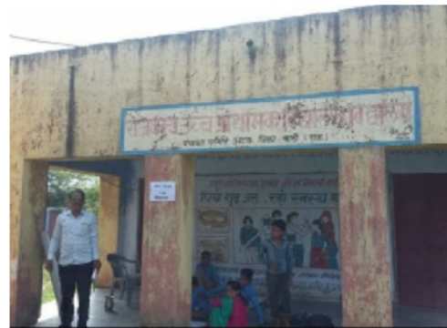
Building Front View
