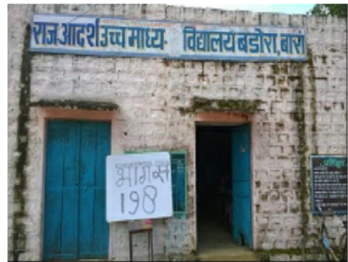
Building Front View
