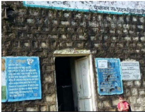
Building Front View
