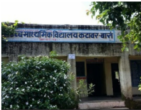
Building Front View
