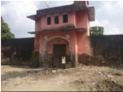
Building Front View
