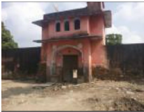
Building Front View
