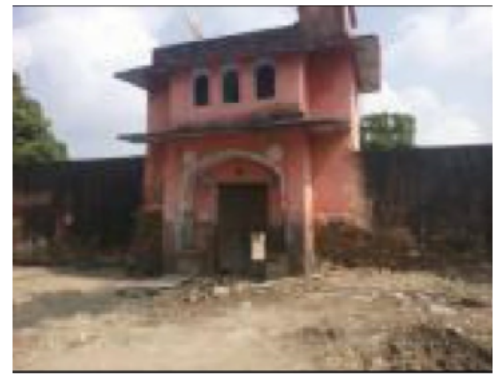
Building Front View
