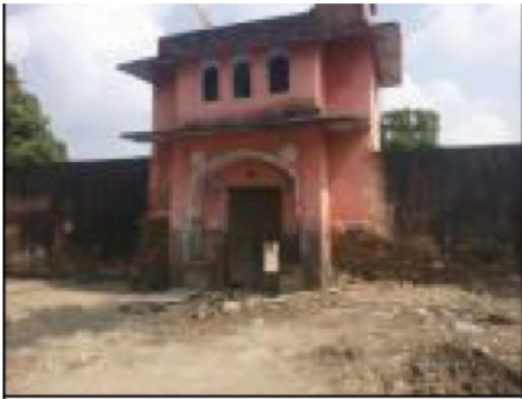
Building Front View
