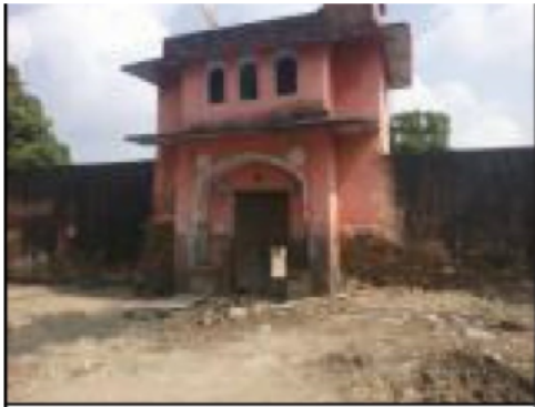
Building Front View
