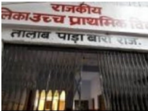
Building Front View
