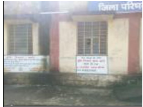
Building Front View
