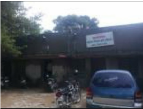
Building Front View
