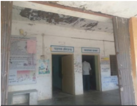
Building Front View
