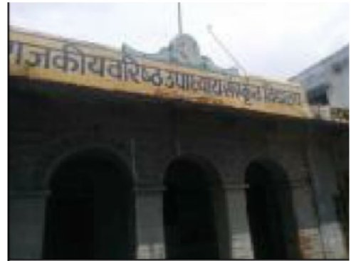
Building Front View
