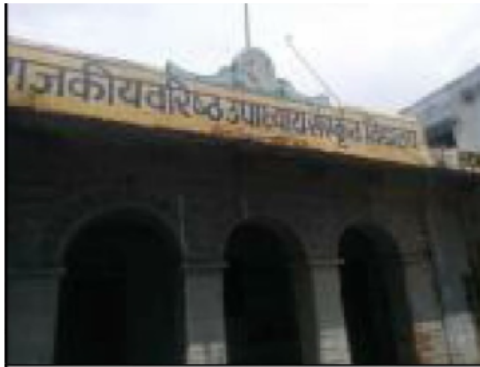
Building Front View
