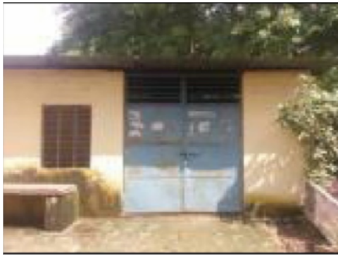
Building Front View
