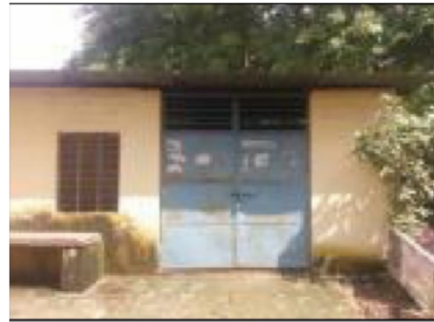
Building Front View
