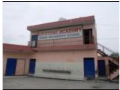
Building Front View
