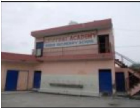
Building Front View
