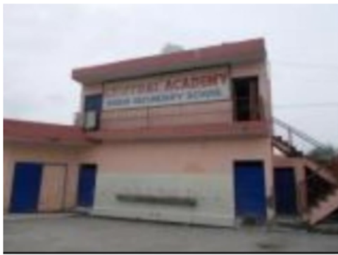
Building Front View
