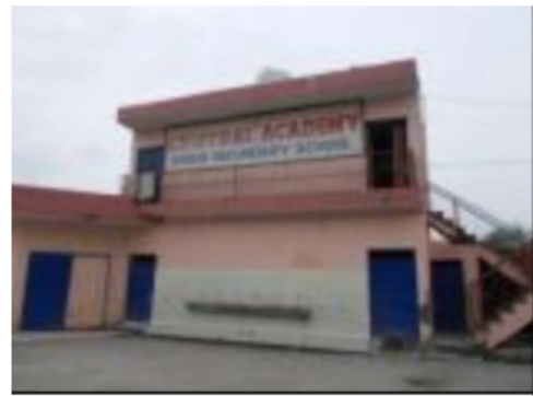
Building Front View
