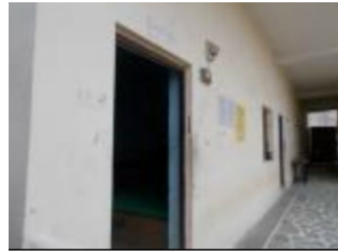
Building Front View
