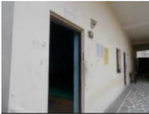
Building Front View
