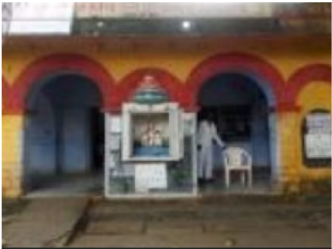
Building Front View
