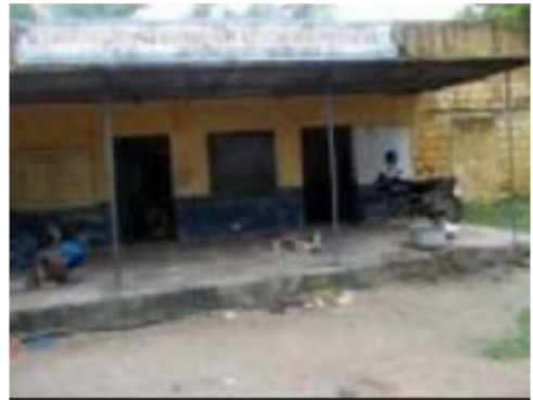
Building Front View
