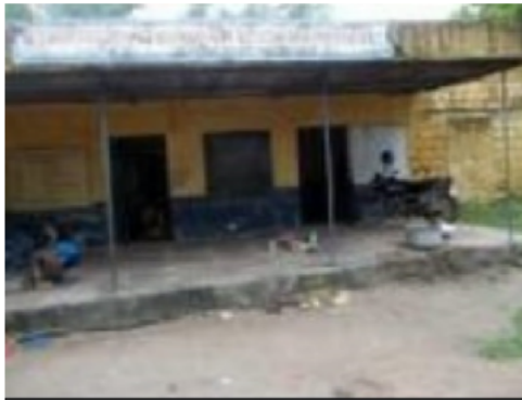
Building Front View
