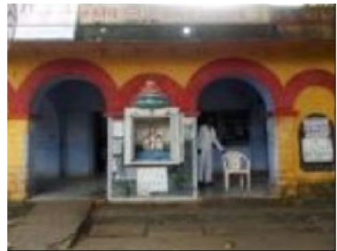
Building Front View
