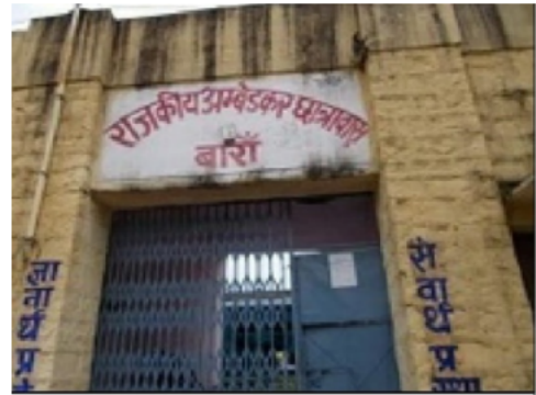
Building Front View
