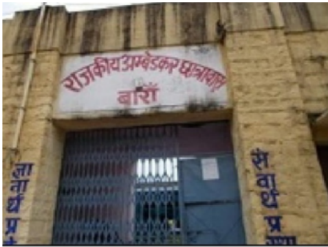
Building Front View
