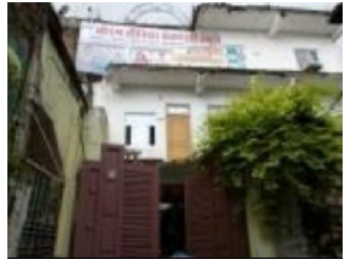
Building Front View
