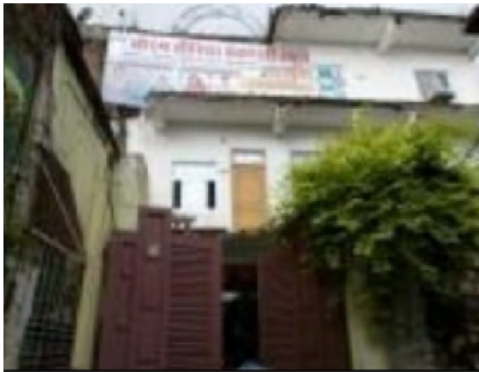
Building Front View
