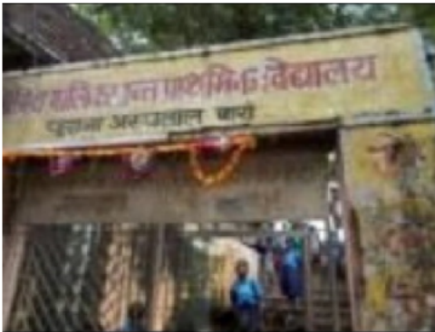
Building Front View
