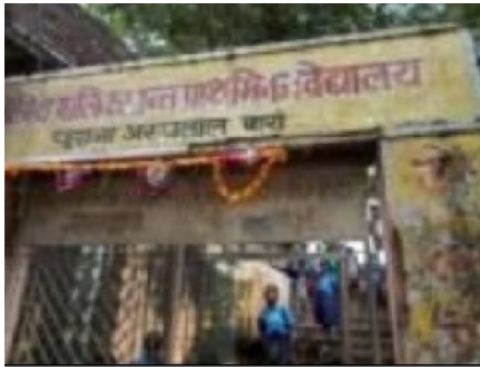
Building Front View
