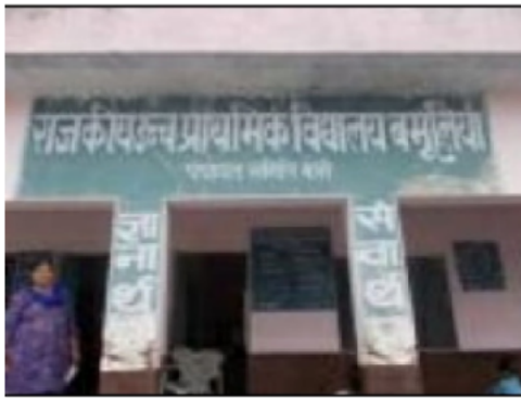
Building Front View
