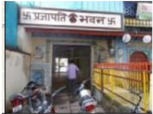
Building Front View
