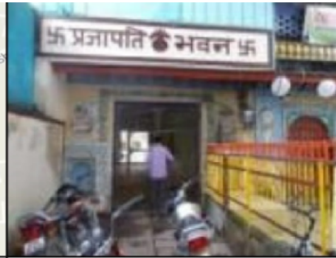
Building Front View
