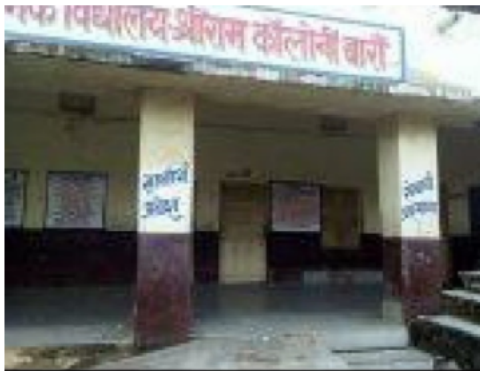
Building Front View
