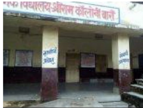
Building Front View
