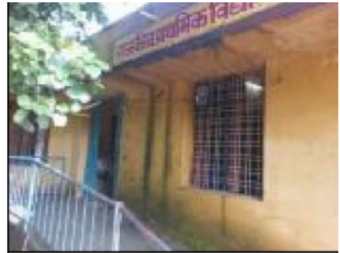
Building Front View
