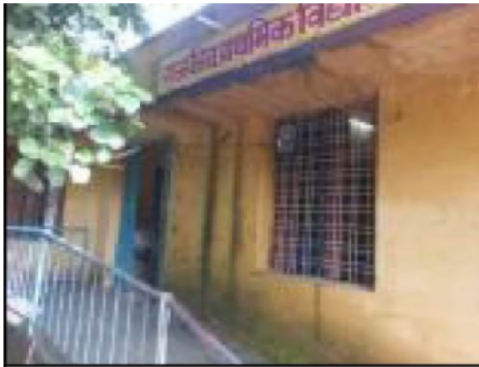
Building Front View
