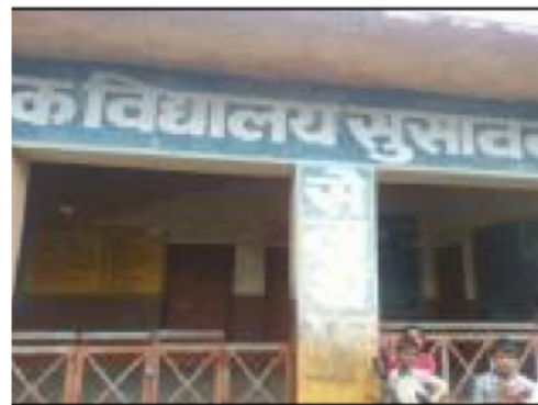
Building Front View
