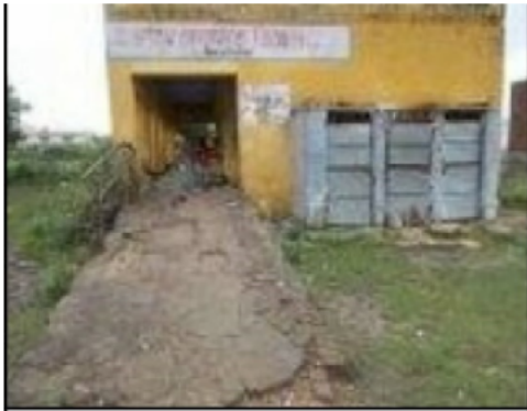
Building Front View
