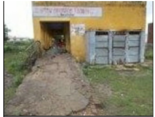
Building Front View
