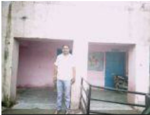
Building Front View
