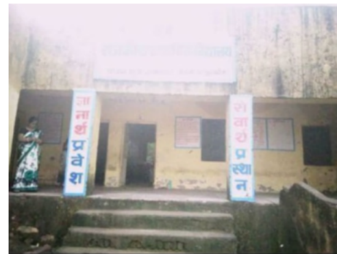
Building Front View
