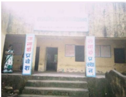
Building Front View
