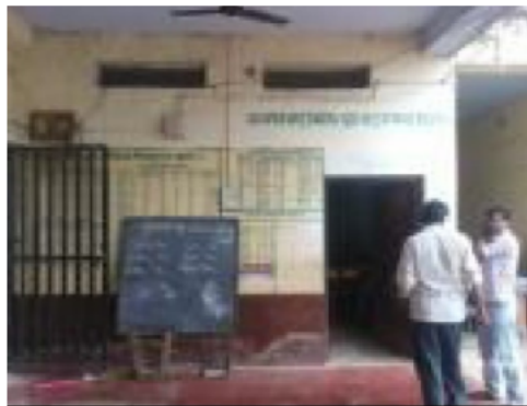
Building Front View
