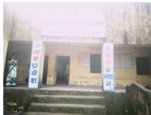
Building Front View
