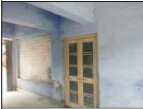
Building Front View
