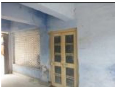
Building Front View
