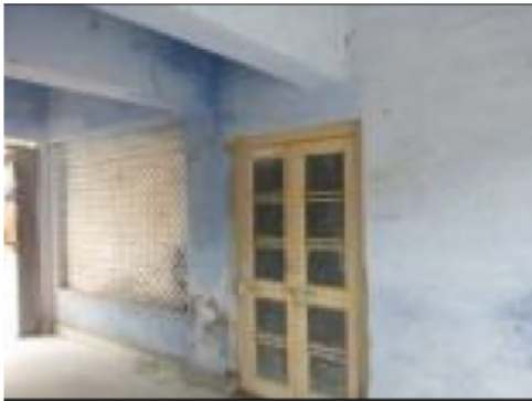
Building Front View
