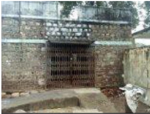
Building Front View
