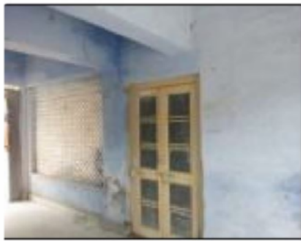
Building Front View
