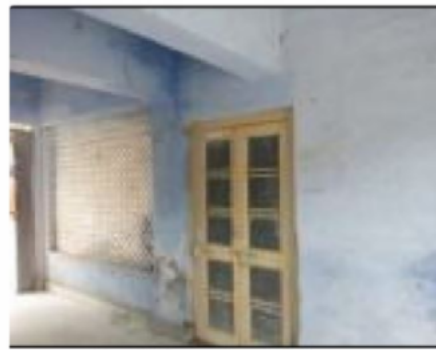
Building Front View
