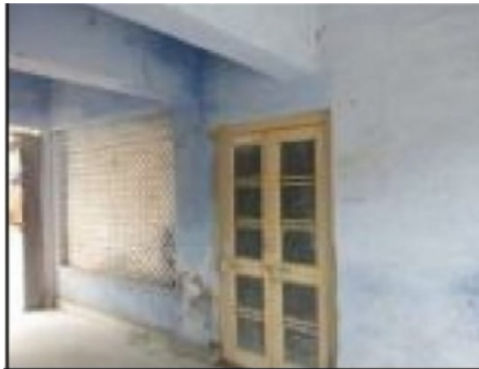
Building Front View
