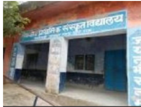
Building Front View
