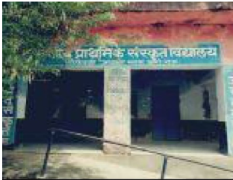
Building Front View
