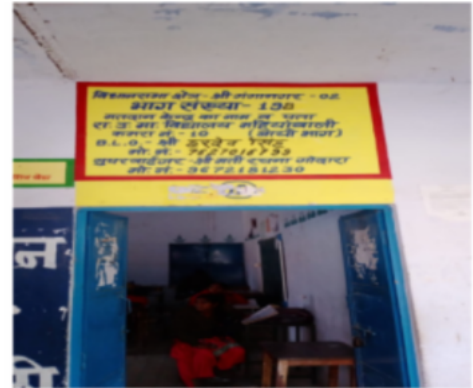
Polling Station Front View
