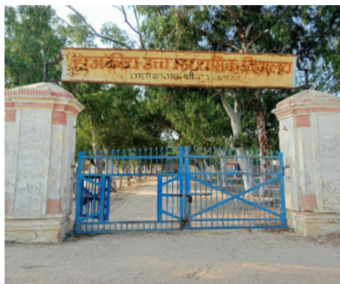
Polling Station Building Front View
