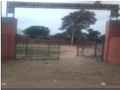
Building Front View
