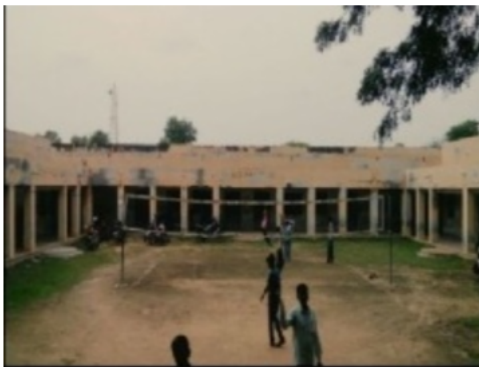
Building Front View
