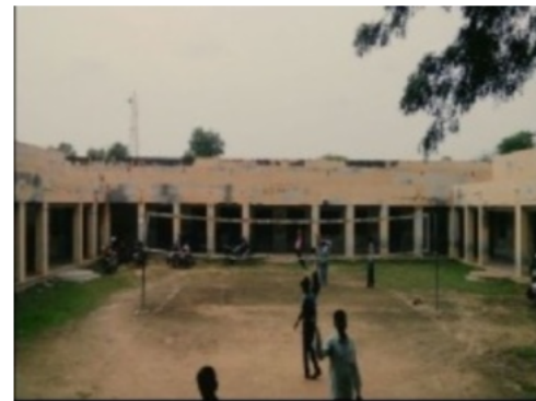
Building Front View
