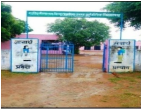
Building Front View
